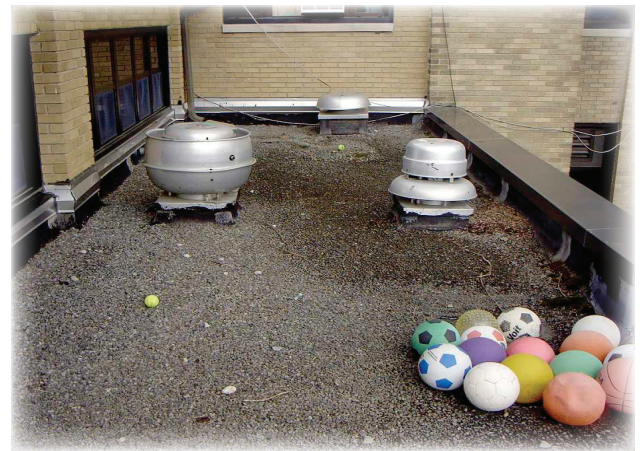
Periodic roof inspections are recommended.
