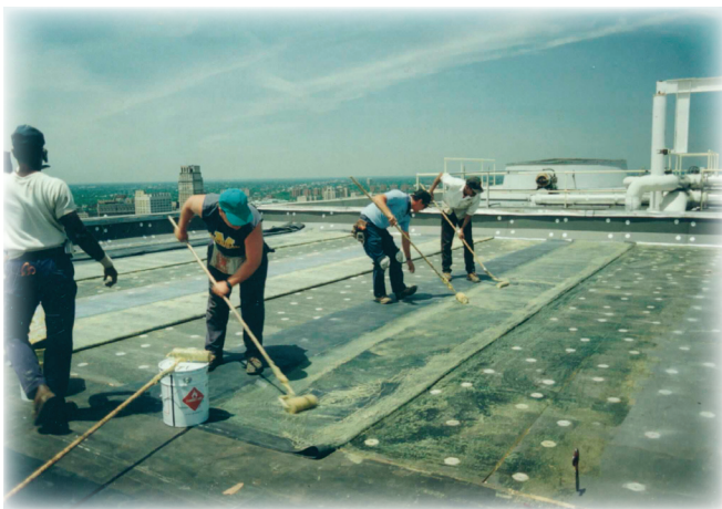
Inspection is the key element for a quality roof.
